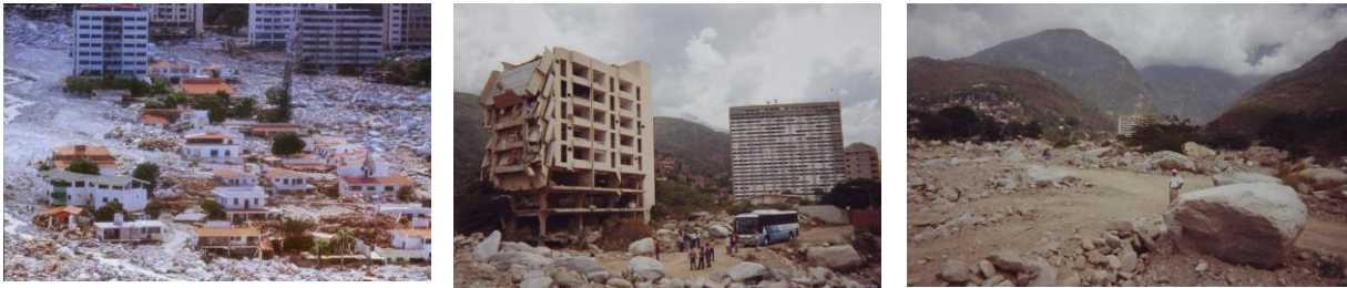
Photo.8 Vargas district along the Caribbean bay coast, near Caracas in Venezuela, was suddenly attacked by unexpected heavy rains in December 1999. After the discussion how to prevent such amount of water and avalanches, the most economic way was to prepare an early warning system for rainfalls instead of heavy concrete protection walls.
