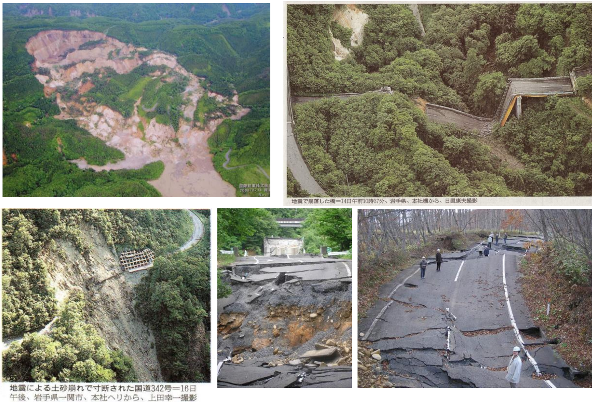
Photo.4 Very large scale land failures happened during the 2008 Iwate-Miyagi earthquake with M7.2 in the northeastern part of Japan. Most of the significant land failures appeared in the area where human developments had been made, such as dams, bridges, mountain roads those had been prepared for the convenience not only for the local people but also for the distant urban people to drive with a shorter ways.
