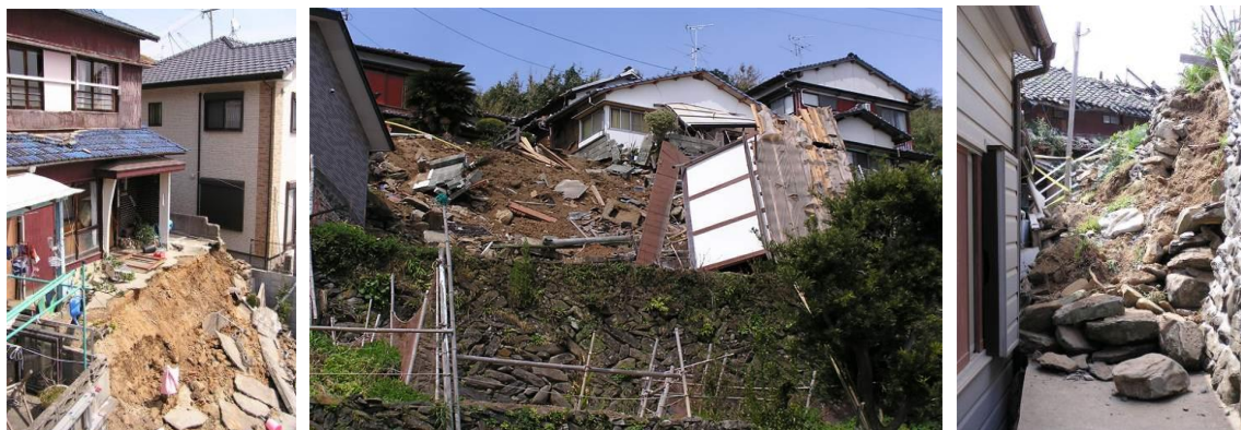
Photo.2 Slope failures those could be seen in a small island near the source region of the 2005 Fukuoka-Oki earthquake. Most of people were fishermen and they preferred daily convenience living near the harbour, then they build their own houses climbing up the slope one and after.
