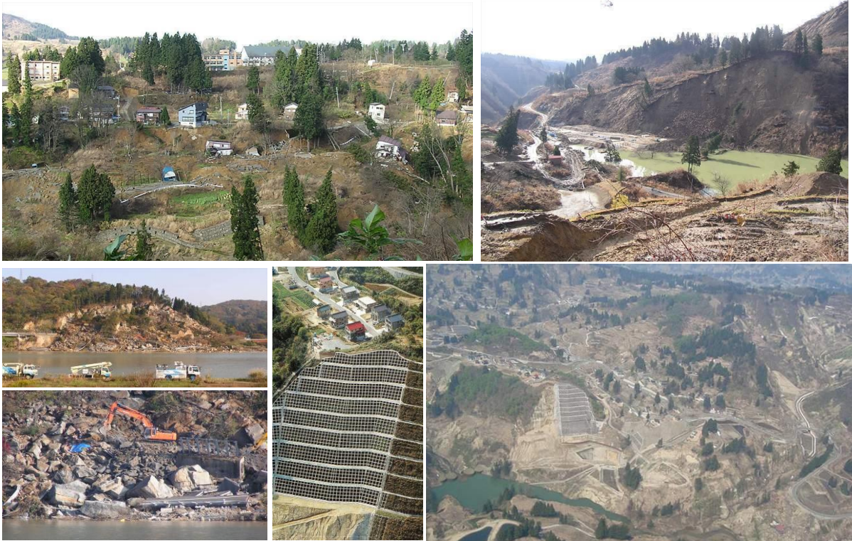
Photo.1 Land failures could be seen everywhere in Chuetsu district in the central Niigata prefecture during the 2004 Niigata Chuetsu earthquake. The most severe damage appeared in Yamakoshi village in the hilly mountain area. It took about three years until the recovery, that means rural residential people came back to their original houses and restarted their daily lives.
