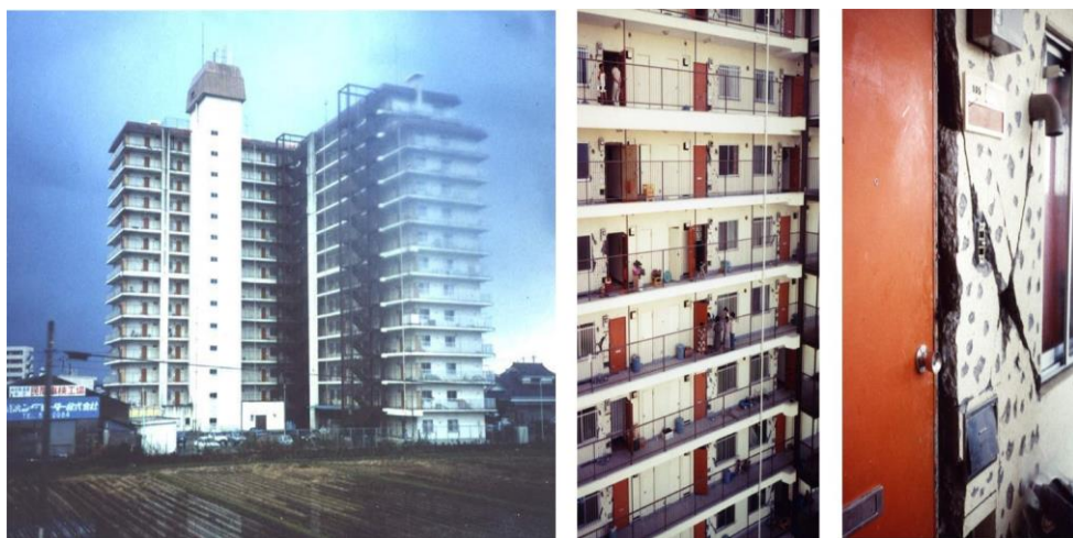
Fig.10 Similar damage had been noticed in the 1978 Miyagiken-oki earthquake in Sendai [1]
